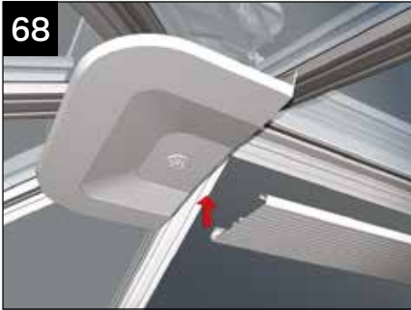
Clip the internal ridge cladding onto the underside of the ridge. In some instances a deep skirt cover may be provided and may need additional trimming on site.
