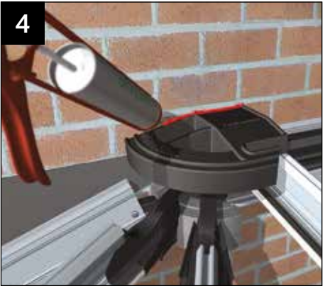
Chase out and install the lead flashing. Add the pre-cut weathering shields. Seal the weathering shield to the host wall.
