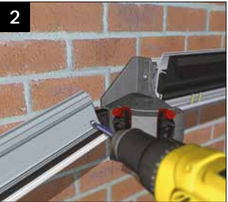
Prior to attaching the starter bar to the mounted starter bar bracket, remove the M6 taptite screw. Locate the bar on to the bracket and on to the single bolt placed in the eaves beam, re-insert the screw.
